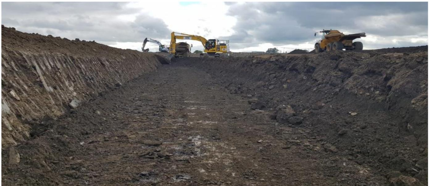
2. Soils arising from the excavation are modified to render their moisture content acceptable for placement as engineered fill in accordance with a density driven specification.
